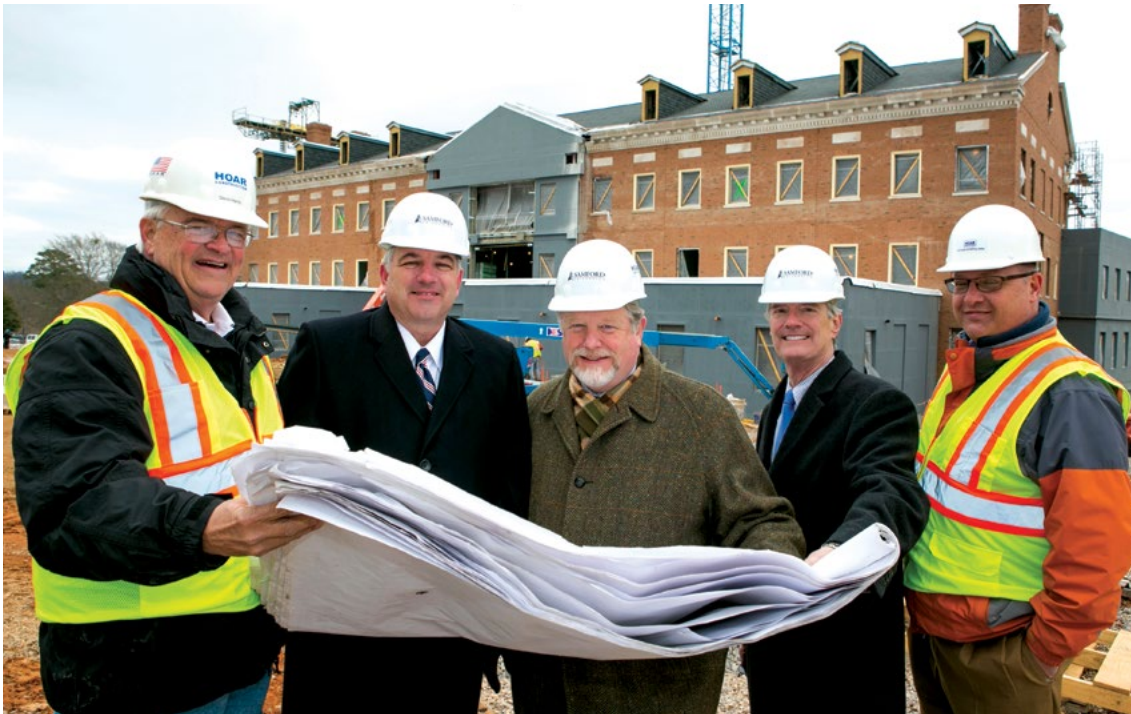
Studying blueprints of the new Brock School of Business Building are, from left, Glen Harris, Howard Finch, Buck Brock, Neil Davis and Mike Waller.
